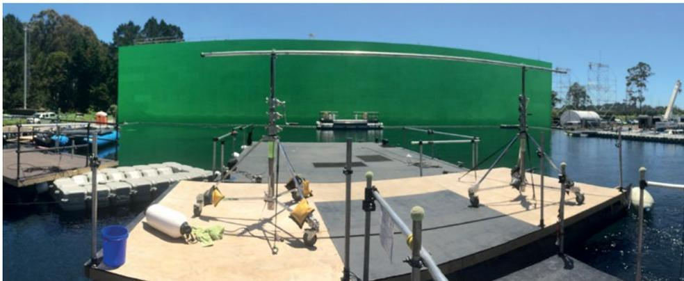
The studios' development for *MEG* included Warner Bros and Gravity funding construction of the first two film studio water tanks ever built in New Zealand: an indoor 5m deep, 1.3 million litre dive tank with pure heated water; and an outdoor 3m deep, 2.5 million litre ocean horizon tank backed by an 864 sq m green screen wall. The studio also has a 4036m<sup>2</sup> sq m stage, production offices, a sought-after forested back lot, and a workshop and manufacturing space.
